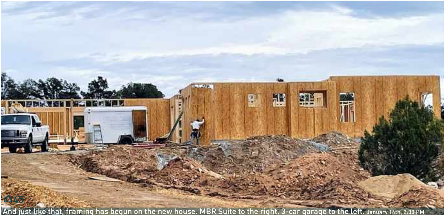
And just like that, framing has begun on the new house. MBR Suite to the right. 3-car garage to the left. January 14th, 2:33 PM
