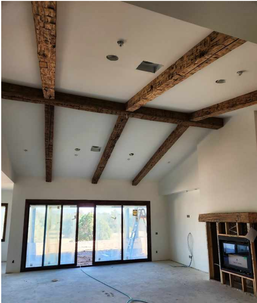
The reclaimed barnwood beams have been installed in the Great Room ceiling and fireplace mantel. Let's hope they are all securely fastened 😊
