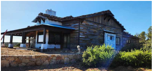
They have completed installing the rustic siding all around the exterior. Next up: the masons will come to cement decorative stone in all the places where you now see white Tyvek. That's Cassie photo-bombing this picture, standing guard over her new backyard.
